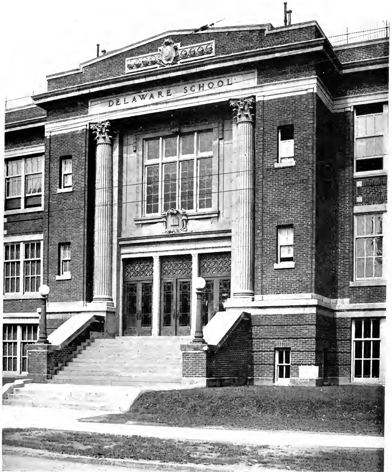
DETAIL OF MAIN ENTRANCE DELAWARE SCHOOL, SYRACUSE, NEW YORK JAMES A. RANDALL, ARCHITECT
